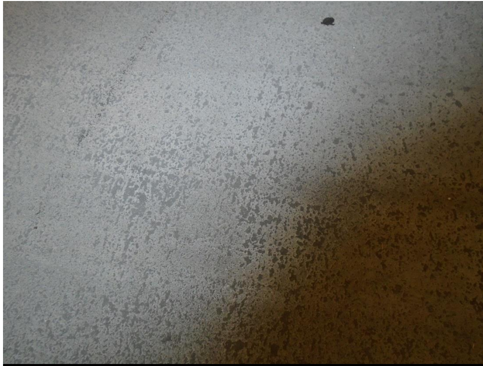
Photo 5. D5 Parking Structure – worn traffic topping.
