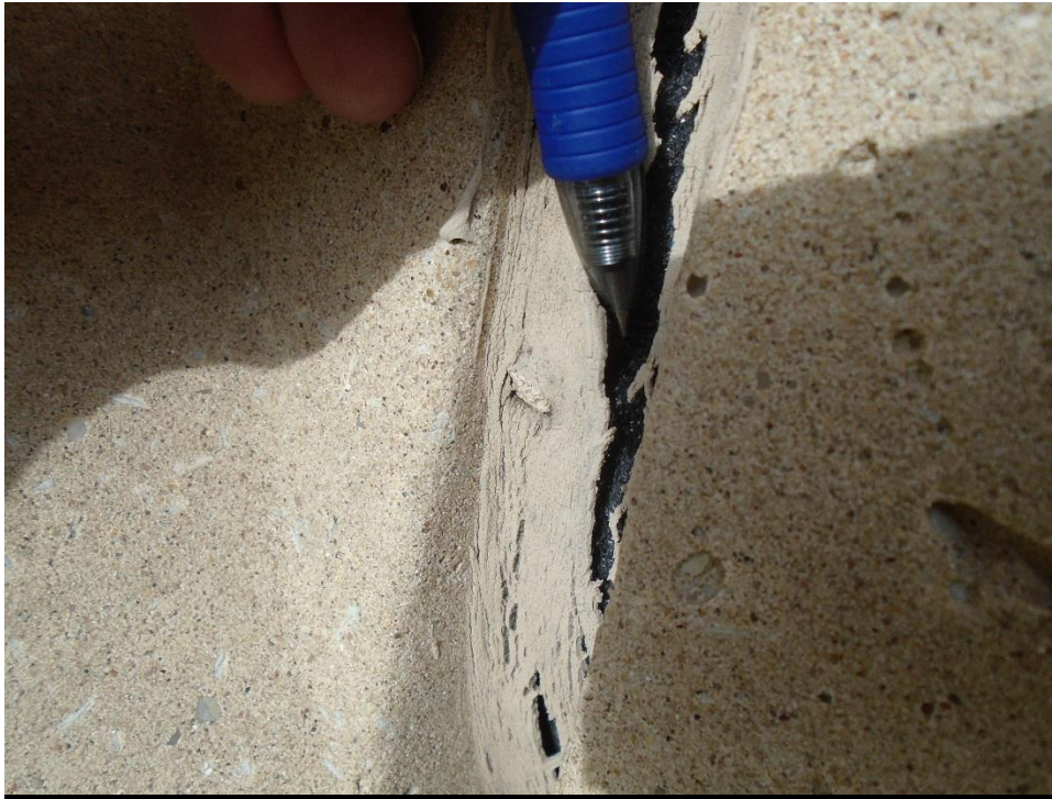
Photo 9. F29 parking structure – failed vertical sealant.
