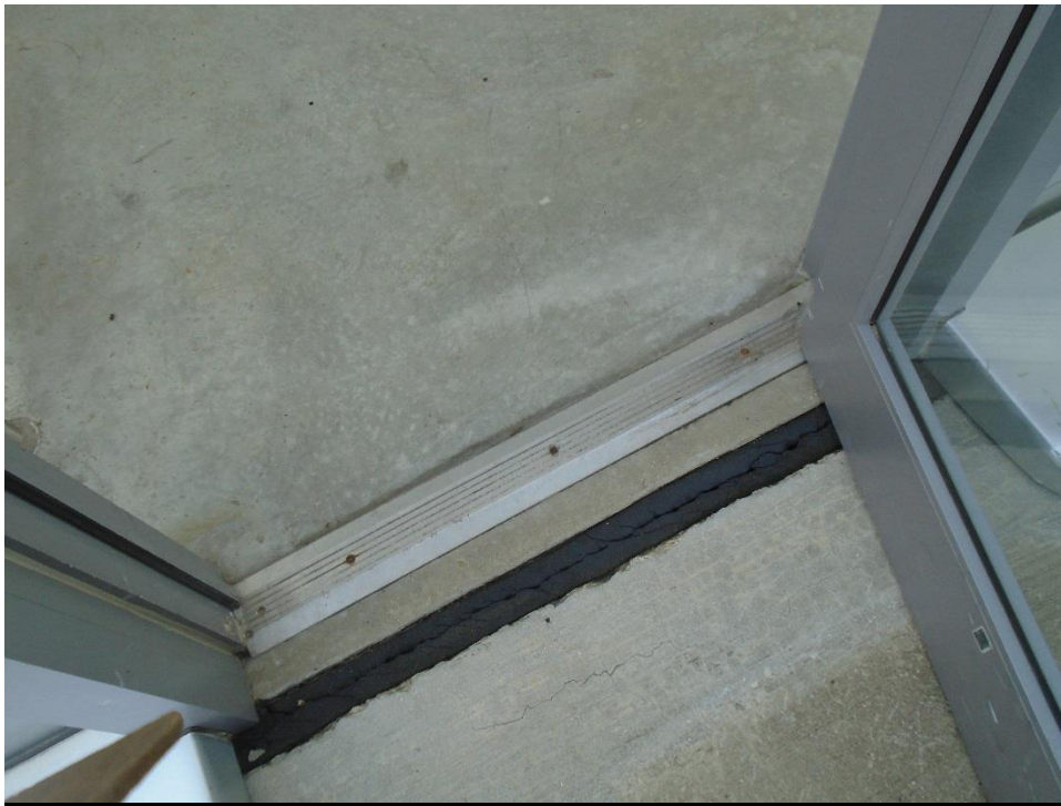
Photo 2. B4 Parking Structure – Failed Stairtower Expansion Joints.
