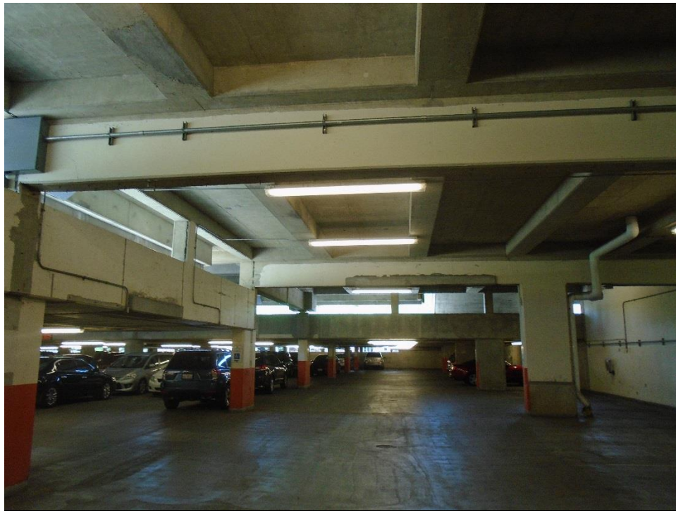
Photo 6. D5 Parking Structure – unpainted locations of previous repairs.
