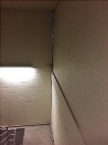
Bioprocess Laboratory: Structural wall crack
