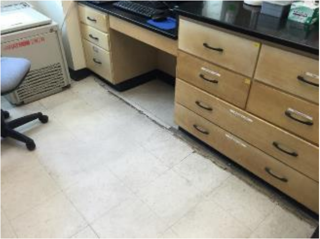
Madigan Laboratory: Structural slab settlement
