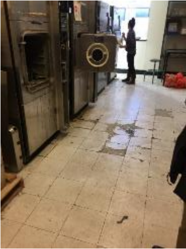
Madigan Laboratory: Deteriorated floor
