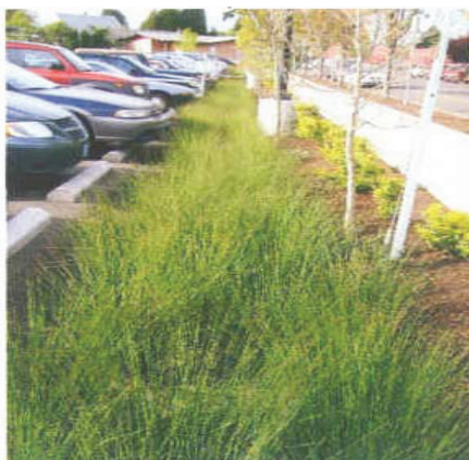
Bioswales: Removing curbs and draining parking towards planting beds can reduce stormwater runoff and increase planting areas to reduce urban heat island effect.
