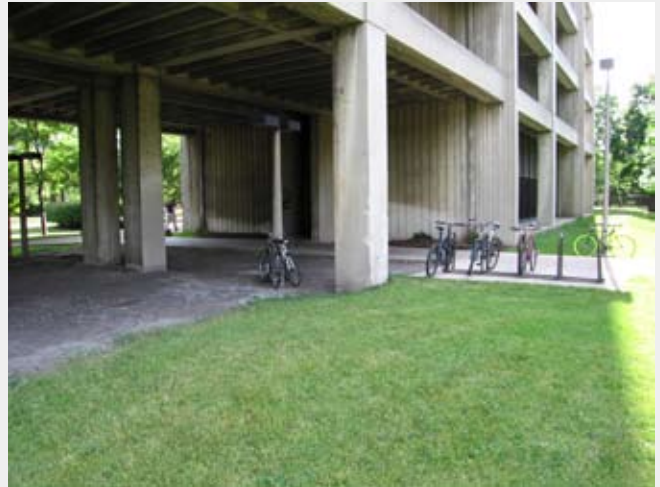
Figure 79.2 Existing building entry enhancement opportunity
