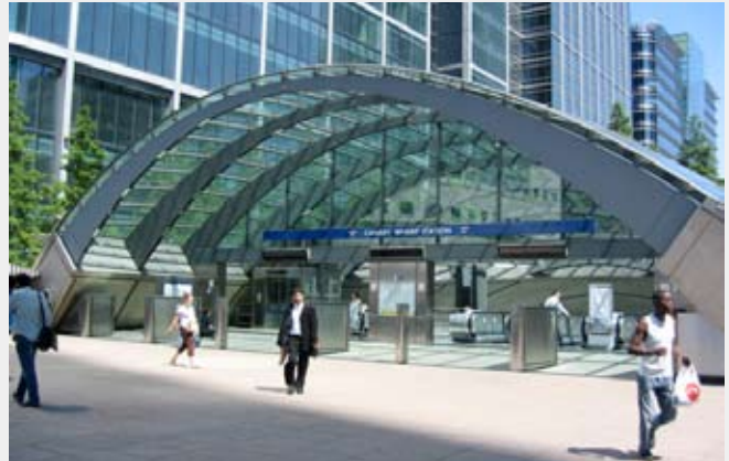
Figure 69.3 Example of transit station entryway
