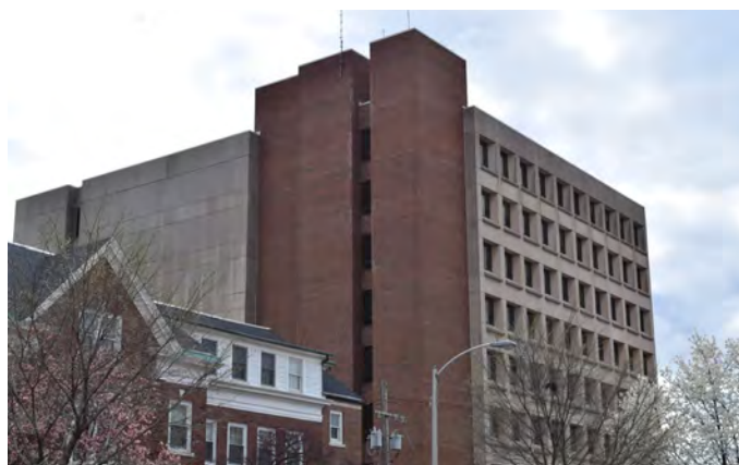
Psychology Building - example of conspicuous elevation in terms of facade's overall vertical proportions
