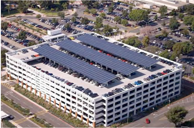
External example of photovoltaic panels on roof of a parking structure
