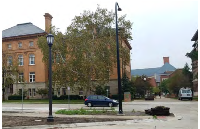
New campus standard fixture to replace historic lantern style fixture
