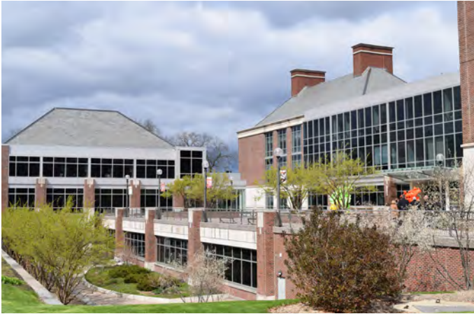
Carl W. Woese Institute for Genomic Biology - roof terrace and courtyard
