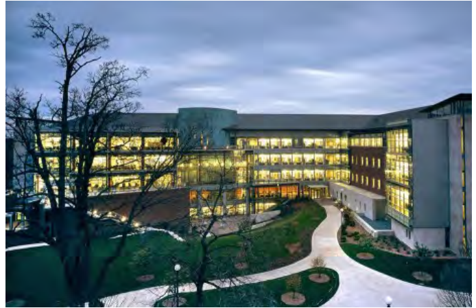
Thomas M. Siebel Center for Computer Science - integrated site design addresses grade issues maintaining accessibility for visitors at the southwest entrance
