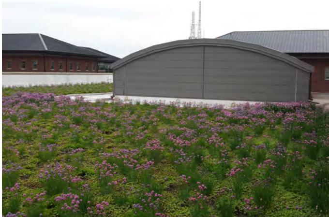
Newmark Civil Engineering Laboratory green roof
