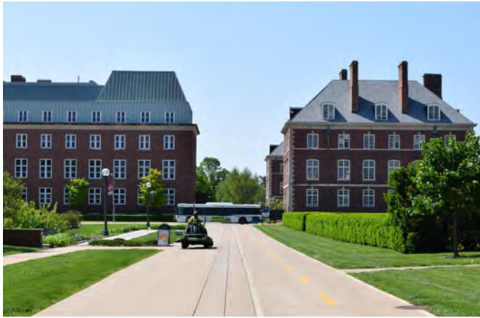
View of Mumford Hall and Animal Sciences Laboratory - example of new roofs relating to existing buildings and composition of stacks and vents at the Mumford Hall
