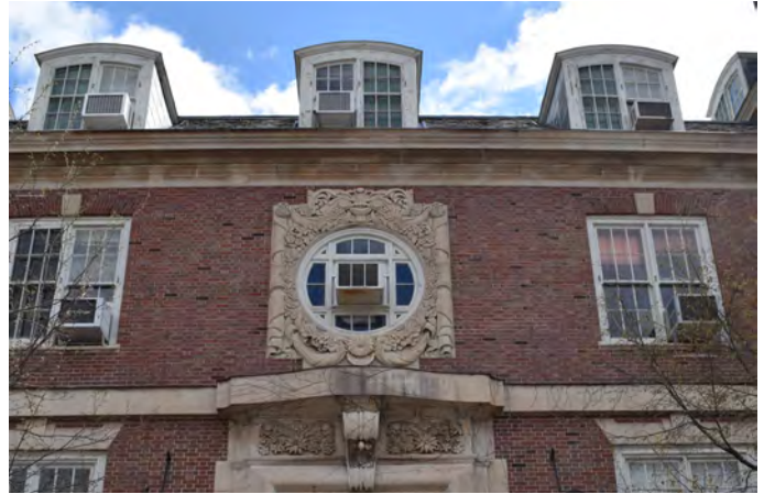
Existing elevation with window air-conditioner units
