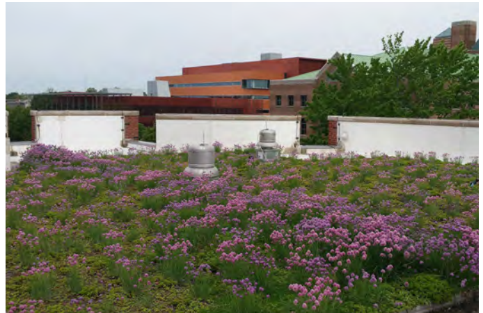
Newmark Civil Engineering Laboratory green roof
